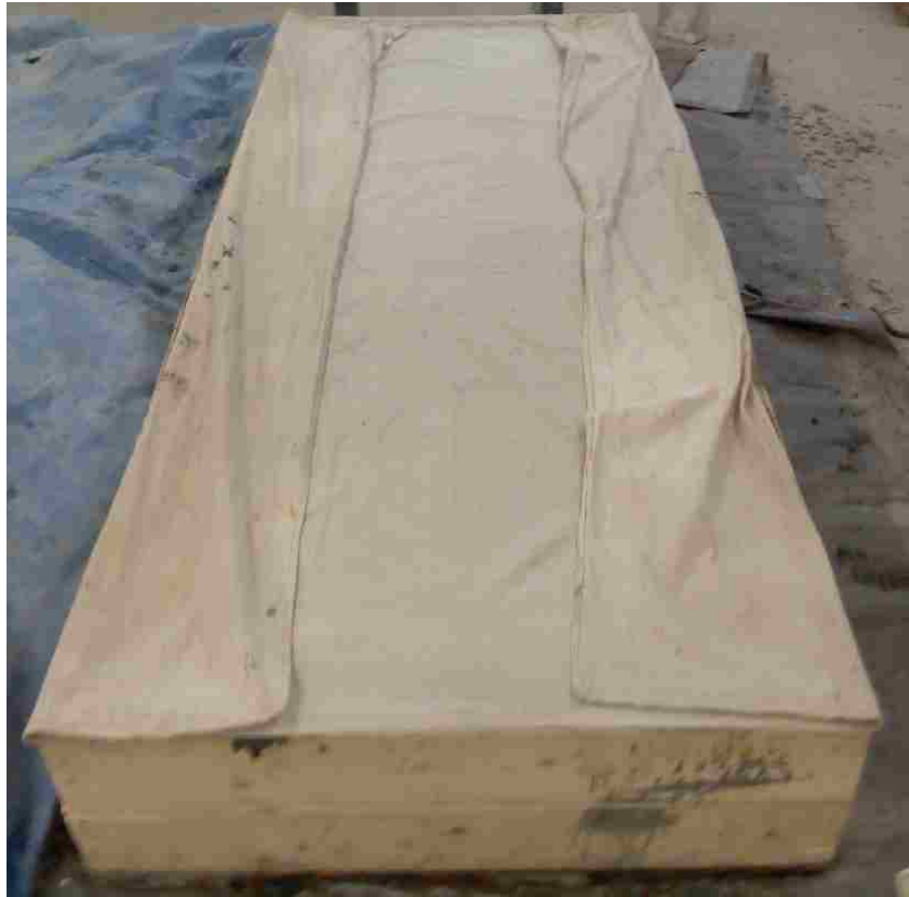
Figure 3.25: Canvas to prevent cracking during the initial set of the UHPC overlay
