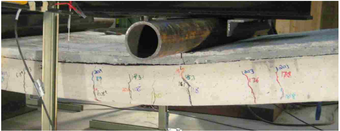
Figure 5.23: UHPC and NVC slab after buckling
