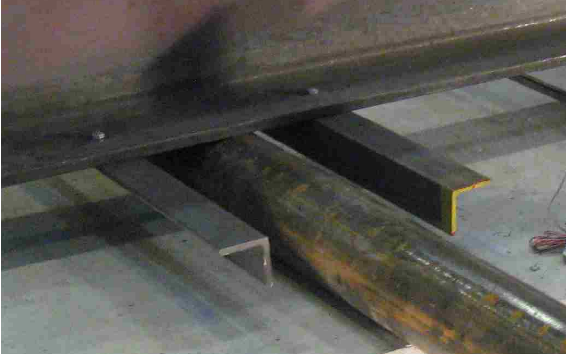
Figure 3.6: Angle iron used to restrict unexpected movement
