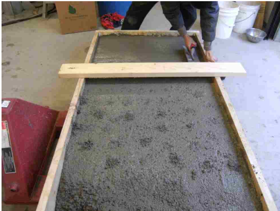
Figure 3.14: Finishing the control slab
