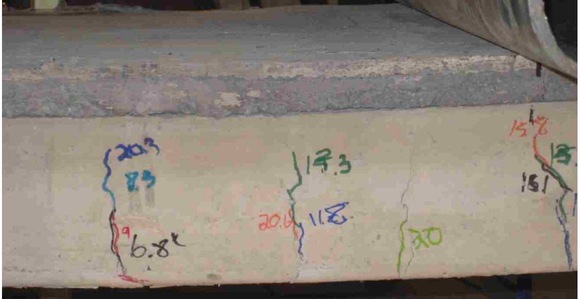
Figure 5.14: Strengthened slab prior to UHPC debonding
