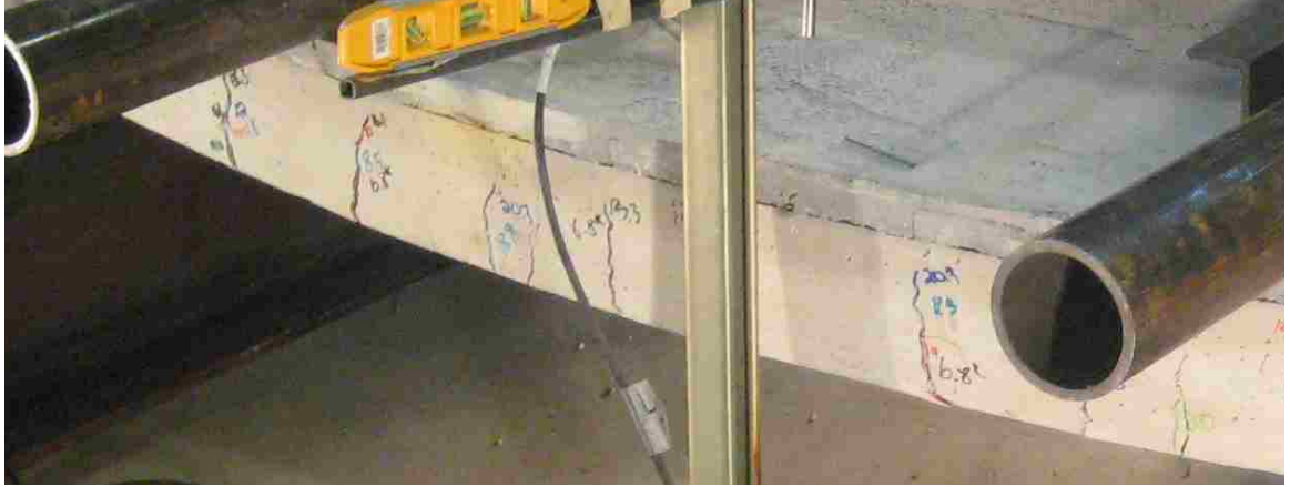
Figure 5.22: UHPC and NVC slab prior to buckling
